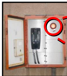
Emergency Trip Station
