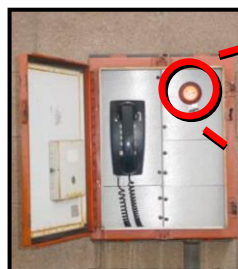
Emergency Trip Station
