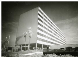
Police Administration Building
