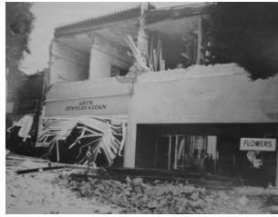
Earthquake damage in Whittier
